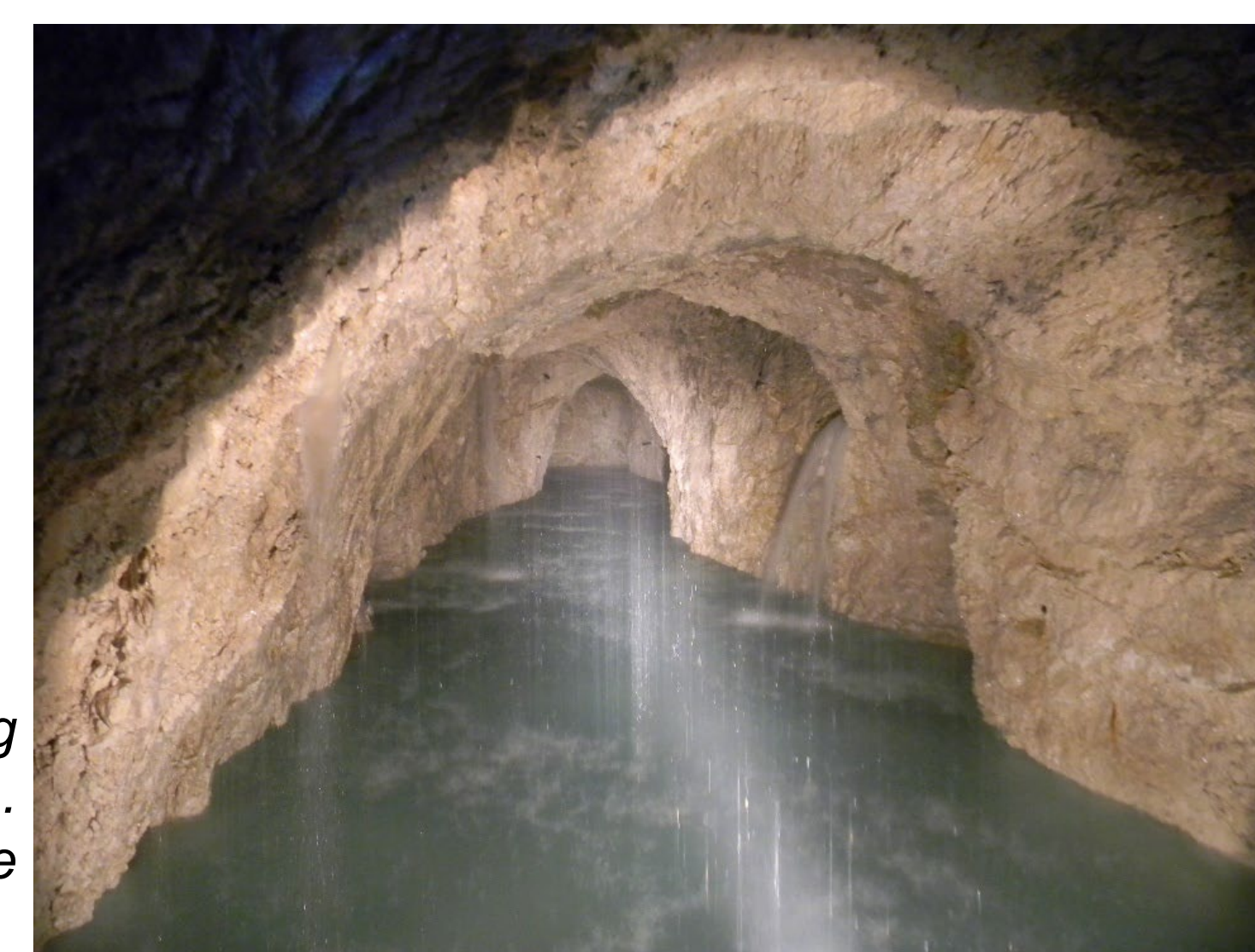
Figure 2. San Chiodo Spring (Umbria-Marche Appennine). Detail of the inner of the water intake structure
