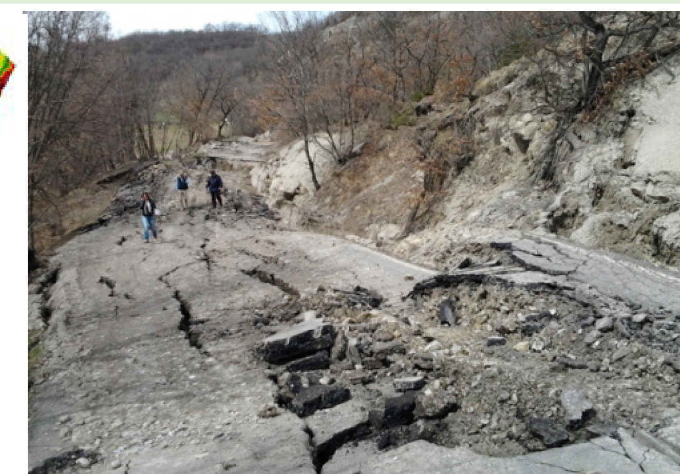
Figure 6. Rotational slide phenomena at Boschetto (Parma).
